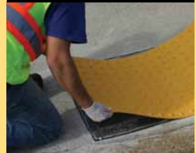
Position the TopMark sheet and hand-tack edges. Clean excess bonder paste from edges.
