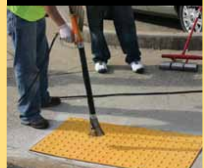
Heat the top surface of the material according to the application instructions.
